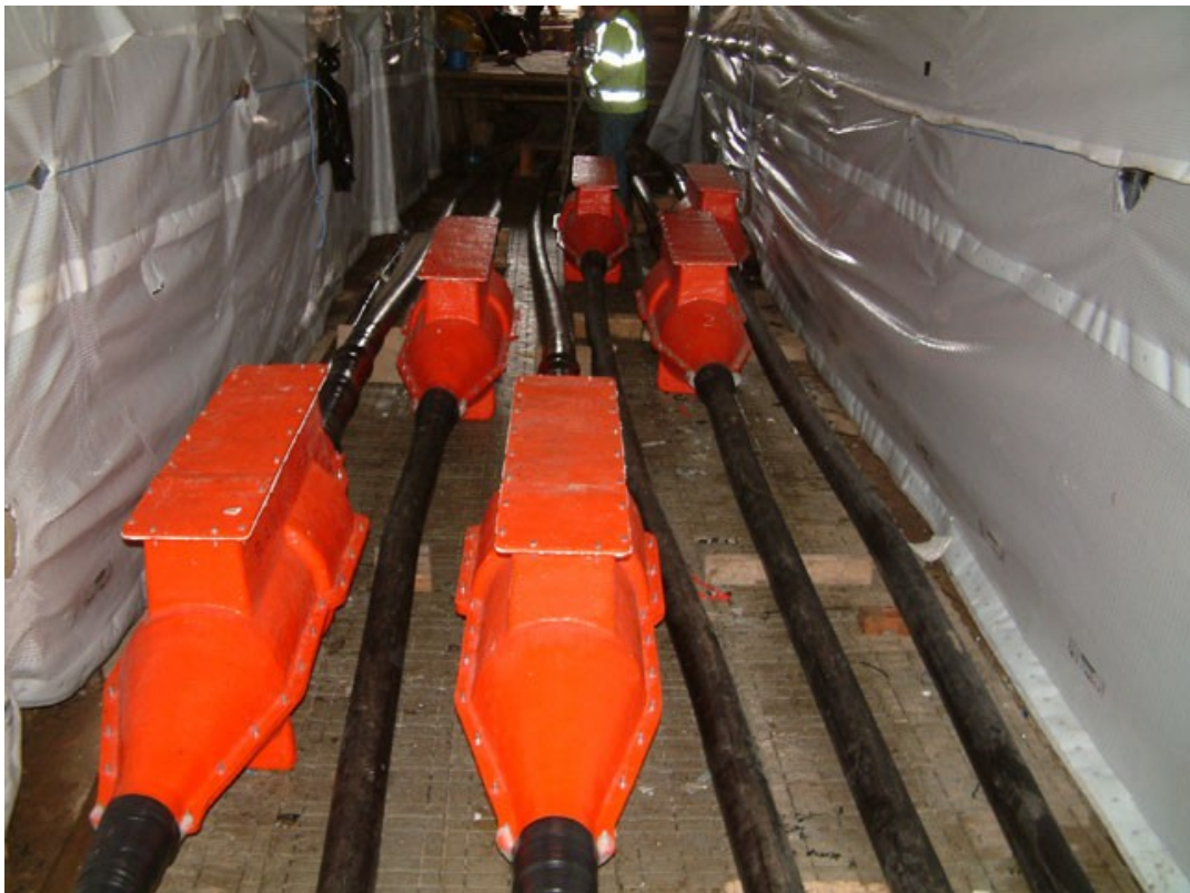
Figure 2 EHV Joint Bay Containing Six Joints
